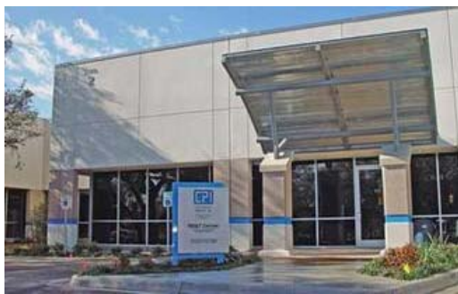
Chatsworth's RD&T Center in Georgetown, TX features several labs and training centers for both customers and employees. Click here to enlarge image
